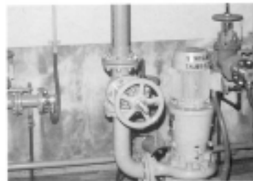
Flange mounting for indoor tank
