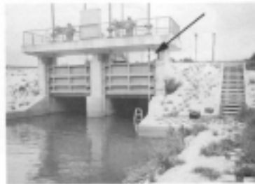
Open angle control of the rever gate (The PL is in the stilling tube)
